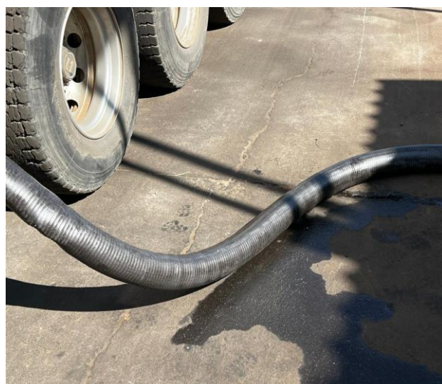
Picture B: Leaking offloading pipe.
