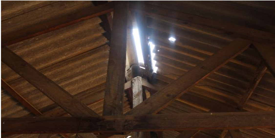
Picture 6: Leaking flea market roof for Makonde RDC.
