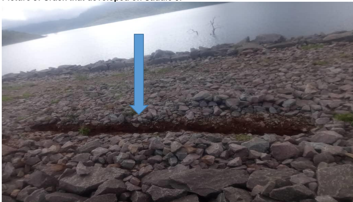
Picture J: Crack that developed on Saddle 3.
