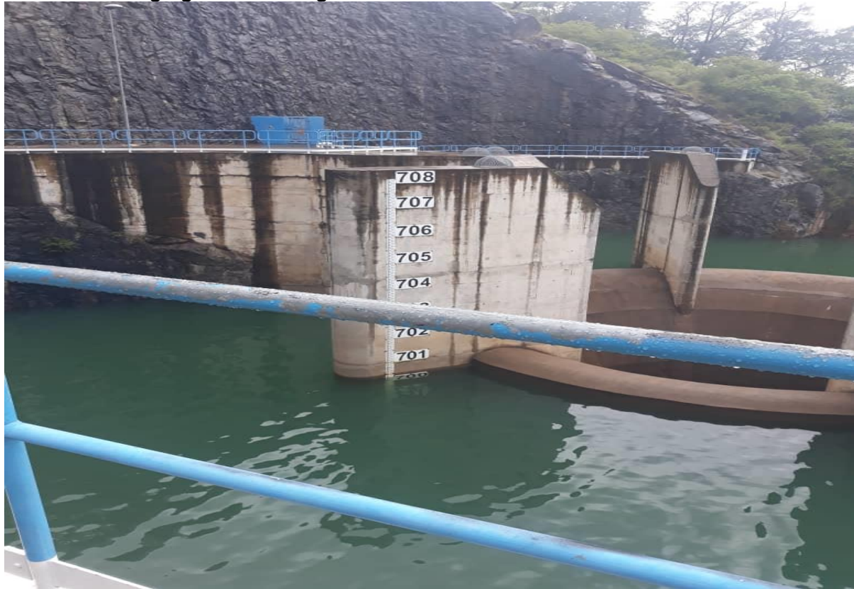
Picture K: Gauging Plates at Tugwi Mukosi Dam.
