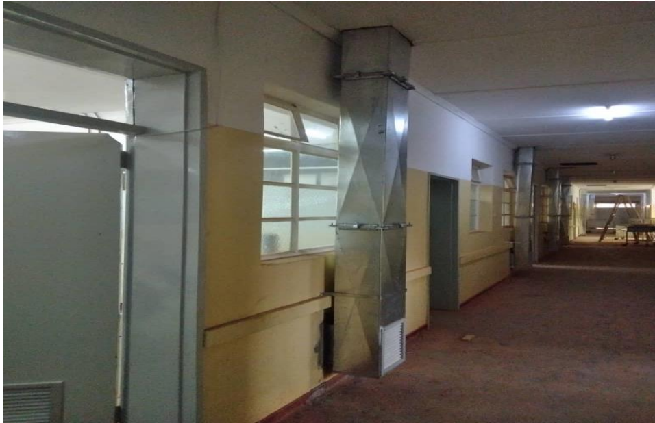
Figure 11: Commissioned Ventilation installed in the Chipinge District Hospital Isolation Centre
