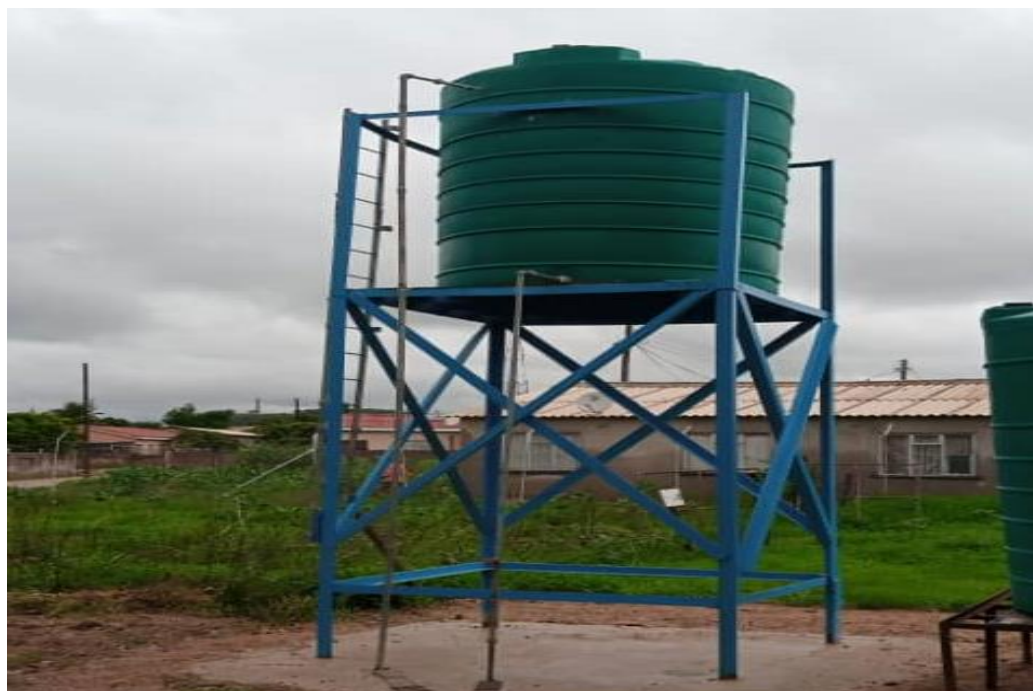
Figure 2: Rujeko Isolation Centre- 5 000 litre tank installed
