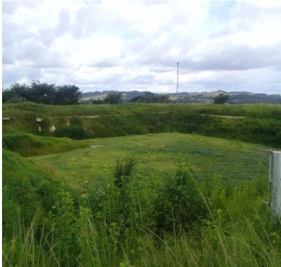
Photo 4- Stabilisation ponds in dire state as they are not being maintained at all
